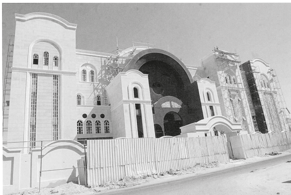
The construction of the new premises of the Coptic Church
